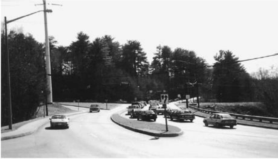
Figure 42 Curbed Island at an Intersection
