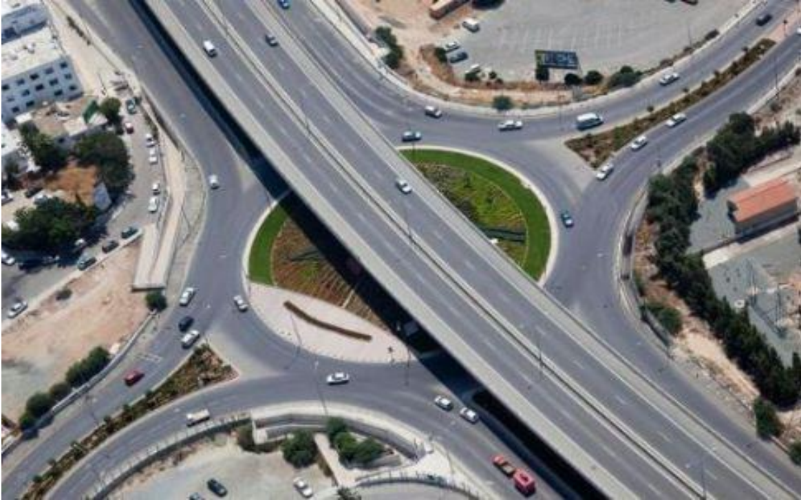
Figure 16 Three-Level Roundabout Interchange
